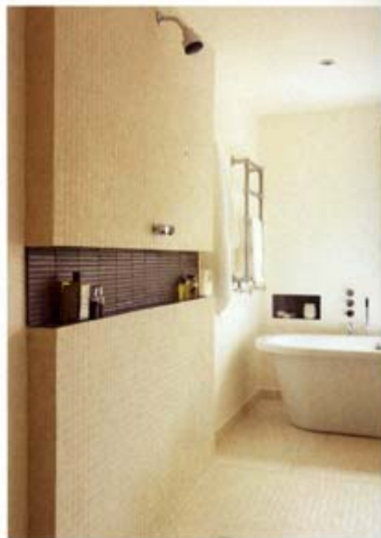
A tiled wall conceals the shower pipework. It also allows for a cut-away section that creates a shelf for shower gels
