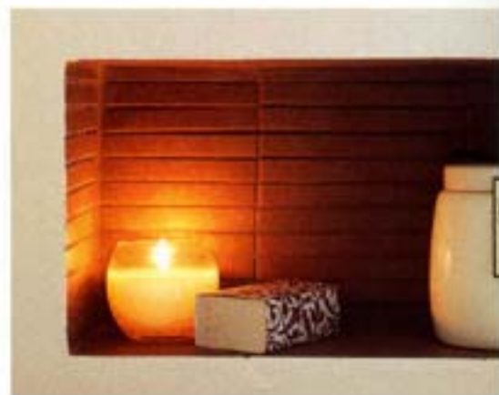
A recess has been cut into the outside wall and tiled in Buxy mosaics to provide a well positioned spot for bath-side toiletries
